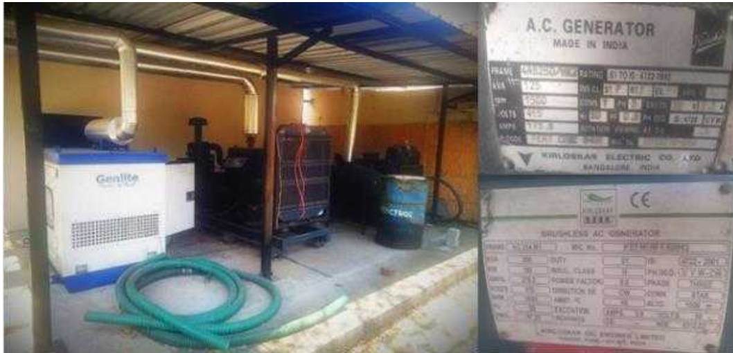
Figure 2.2.3: Diesel Generator Sets & Name plates at JJ College
